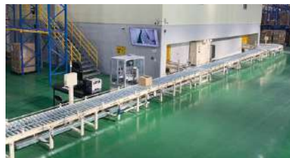
E Plant : E-Beam Irradiation Facility
